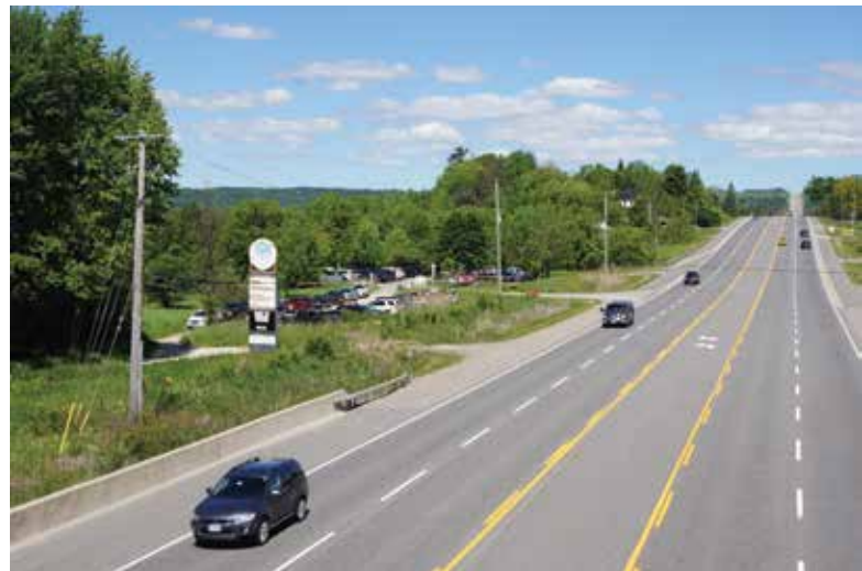
▲ View from the prominent blue bridge that spans busy Highway 10.
