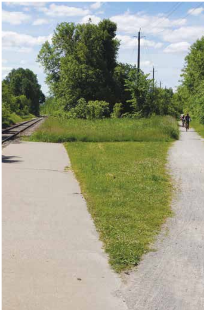
▲ At Inglewood the trail crosses the active rail line, the Orangeville Brampton Railway.
